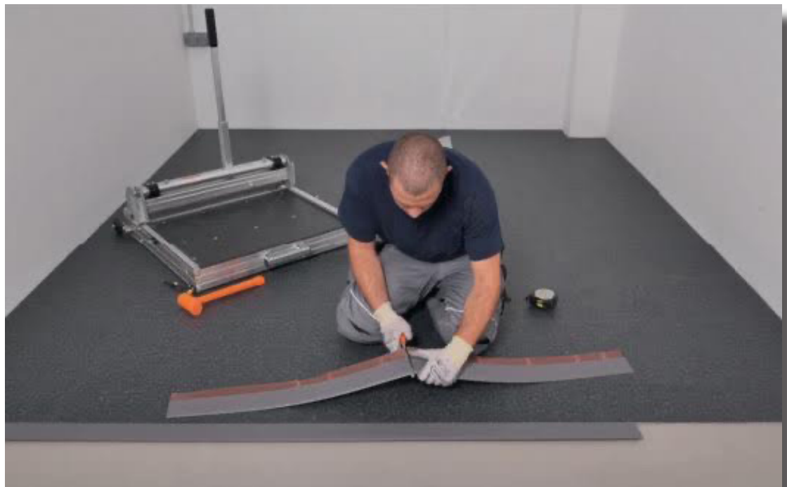
GLUE: Remove protective film from adhesive tape
