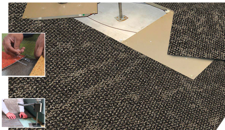
Floating ShadowFX carpet tile installed over access flooring
