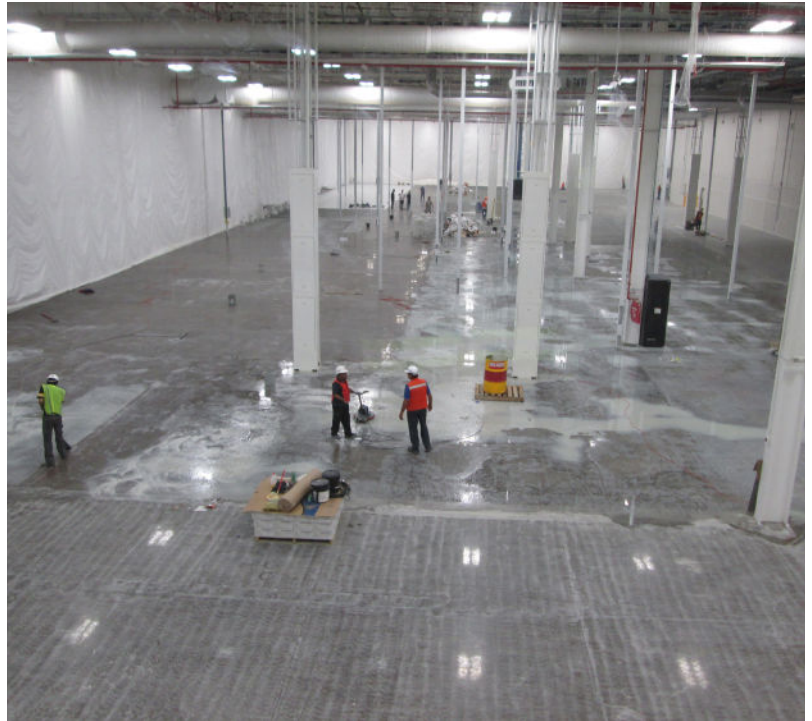
Installation team installing a vapor barrier before laying tile.
